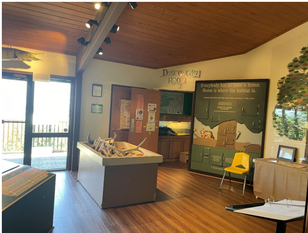
Photo 13: Exhibit Space with open ceiling/exposed glulam structure and decking. Entrance to Discovery room from exhibit space.
