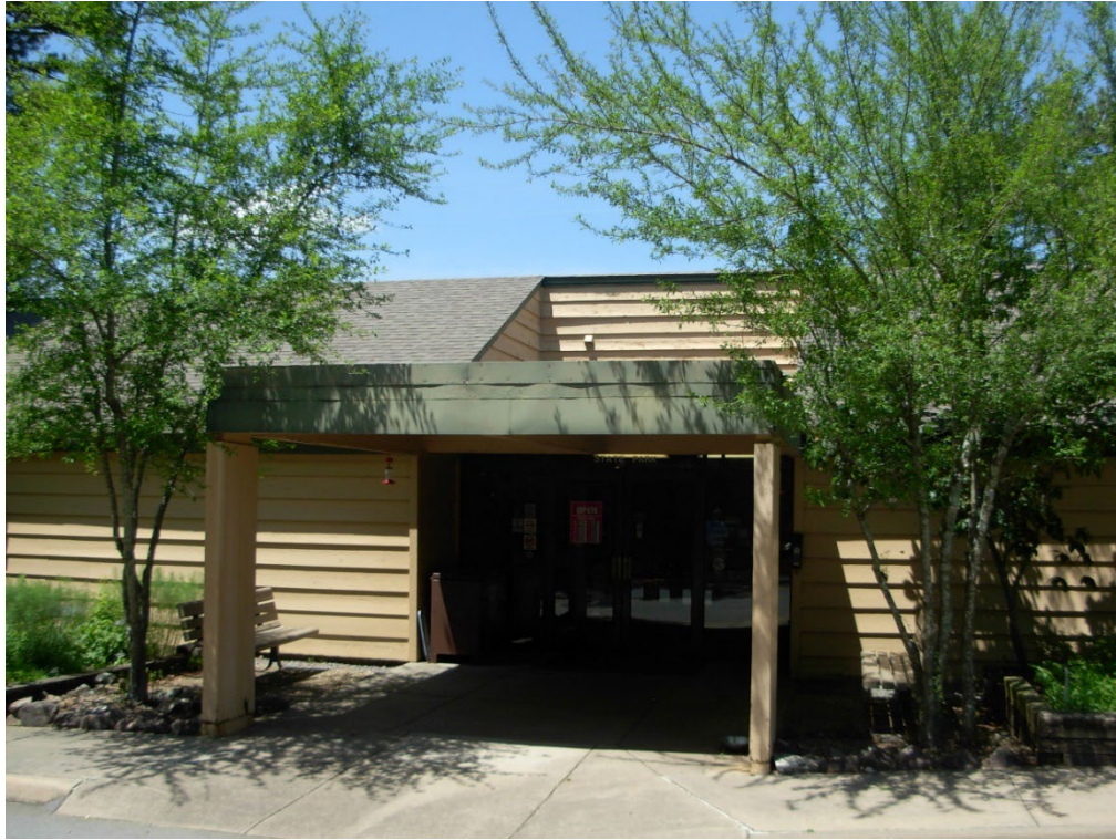
Photo 1: Front (South) Entry Overview. The wood siding is decayed and has been damaged by animals and insects. The metal fascia on the entry is warped. Owner noted drainage issues at flat roof.
