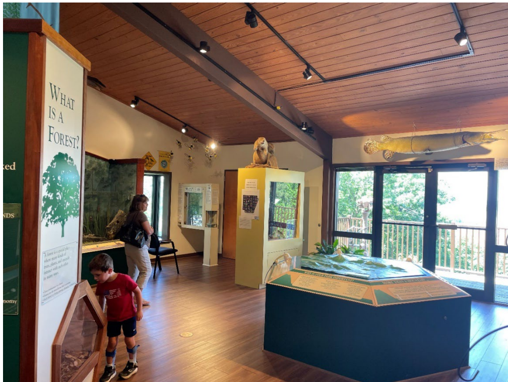
Photo 12: Exhibit Space with open ceiling/exposed glulam structure and decking.
